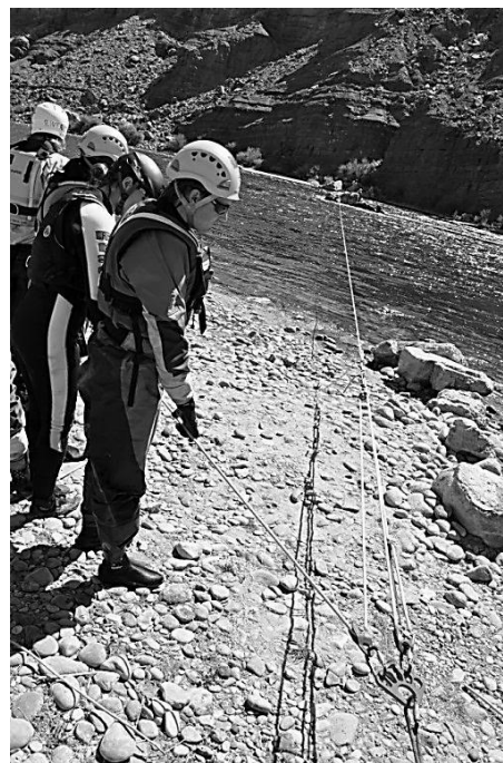
FIGURE W75. Rescuers remain outside the bight formed by a mechanical advantage system and on the upstream side of the line. This practice protects rescuers in the event equipment failure and the sudden forces that could be dissipated.
