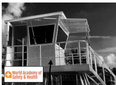
Lifeguard tower for one or multiple lifeguards. Used in select geographic areas and can be equipped with telephones, climate control, polarized windows & more. FIGURE C.7.2
