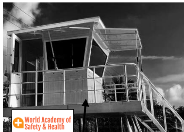
Lifeguard tower for one or multiple lifeguards. Used in select geographic areas and can be equipped with telephones, climate control, polarized windows & more. FIGURE C.7.2
