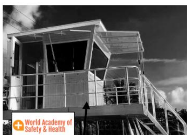
Lifeguard tower for one or multiple lifeguards. Used in select geographic areas and can be equipped with telephones, climate control, polarized windows & more.
