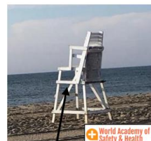
Lifeguard chair for a single lifeguard. It is elevated above the level of the swimmers and far enough behind the high tide line that it is not washed away or damaged by the incoming tidal flow and/or wave action.
